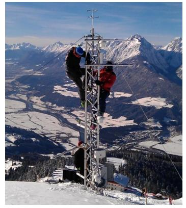
Figure 1. Preparation for the TEAMx Observational Campaign: work on one of the long-term surface energy balance towers in highly complex terrain in the Inn Valley Target Area, Austria, one of three target areas in TEAMx. Photo courtesy of Ivana Stiperski, University of Innsbruck.
